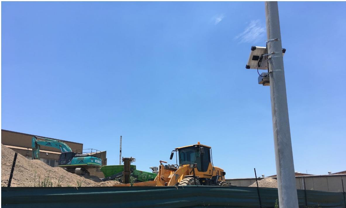
A low-cost particulate sensing device installed to monitor dust arising at the construction site, Parramatta, NSW. Image source: UTS
