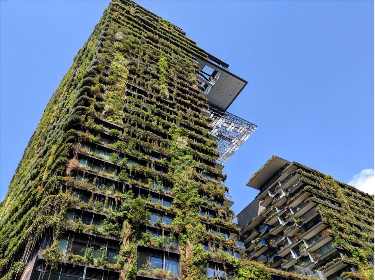
Green walls like this one in Central Park, Sydney (NSW) can actively clean pollutants from the air. Image source: Creative Commons
