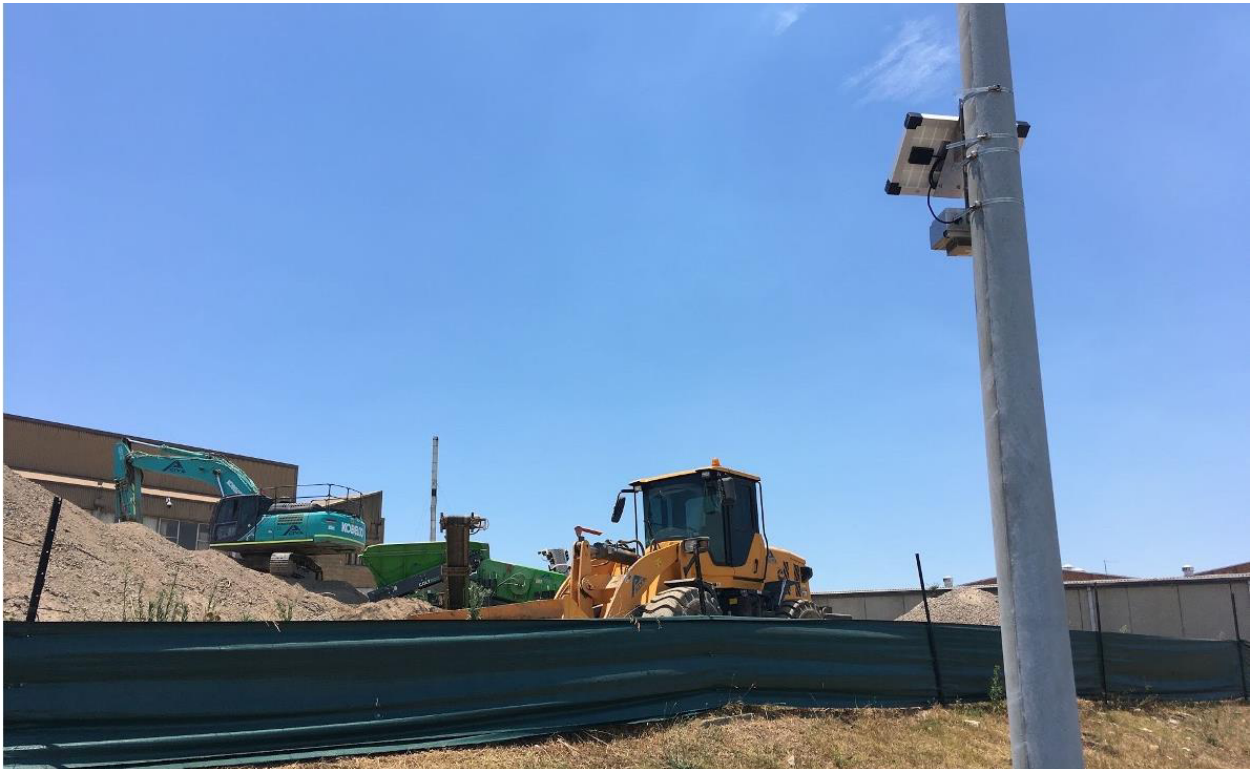
Sensing devices installed to monitor dust at a construction site in Parramatta, NSW. Image source: UTS
