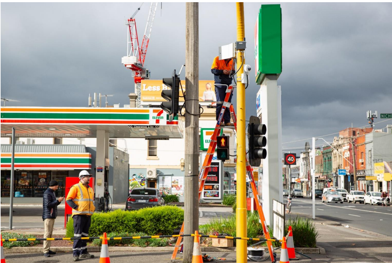
Smart traffic lights being installed in Fitzroy, Victoria. Image source: Cesar Nicolas, University of Melbourne
