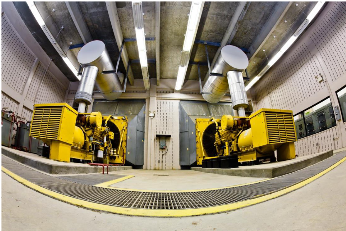
Most commercial buildings have at least one backup generator in their basement, and larger buildings may have several.
