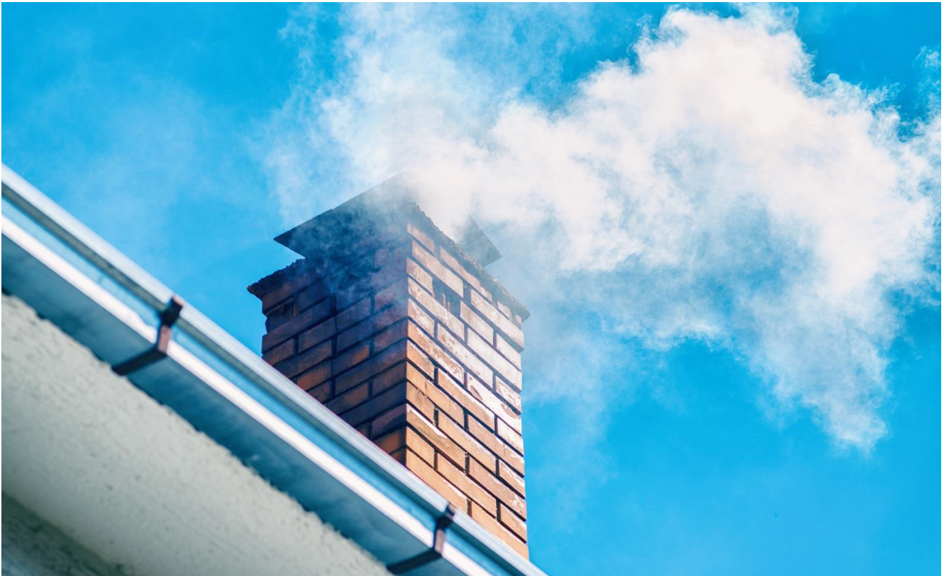
Wood smoke from domestic heating can be a major source of urban air pollution.
